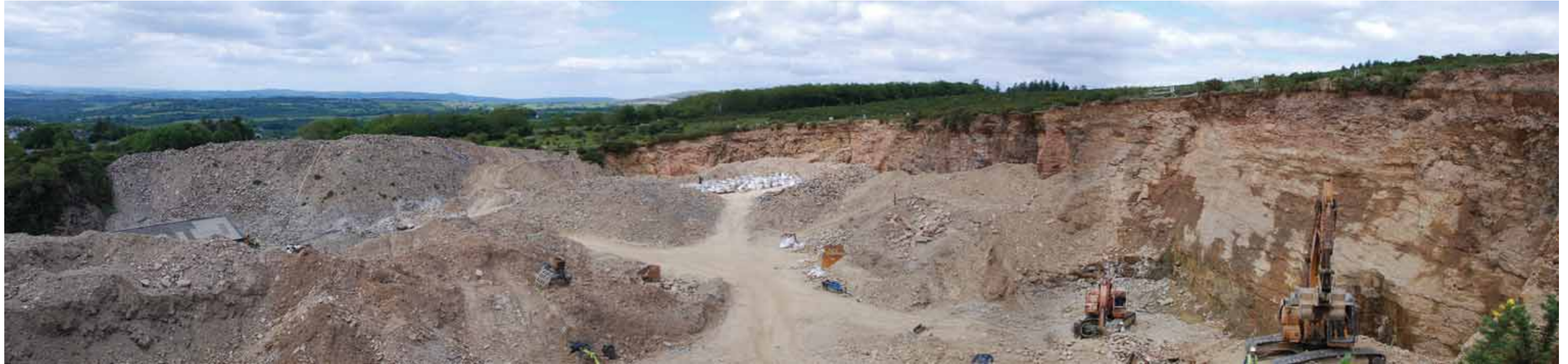
Site Photograph L: Looking north into the existing working area in the south eastern corner of the Quarry
