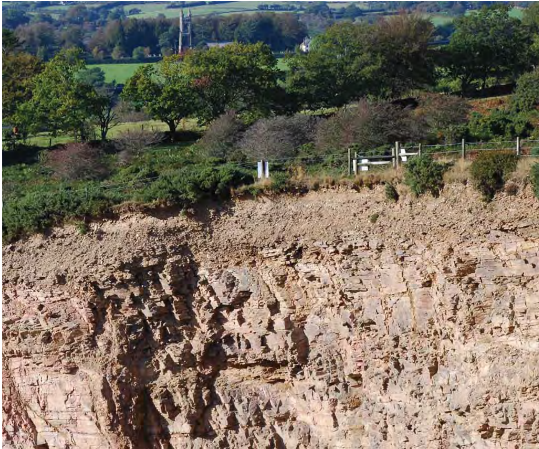
Site Photograph S: Looking east towards the existing northern face of the Quarry
