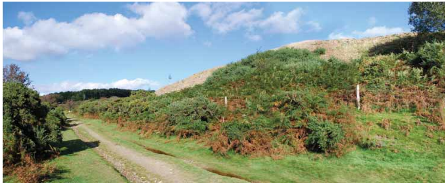
LVA Photograph 2: Looking north along the western boundary of the Site towards existing Screen Bund
