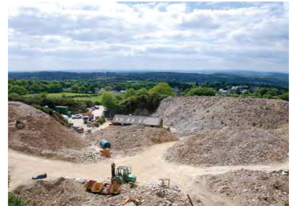
Site Photograph I: Looking towards Processing Area
