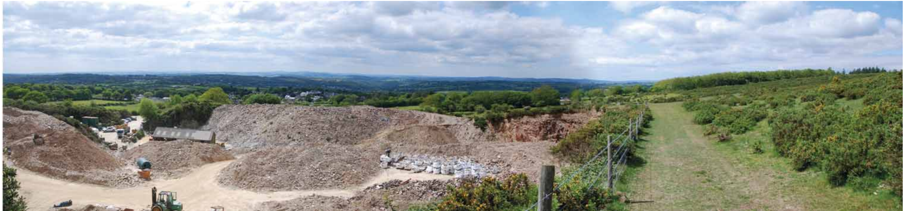
Site Photograph J: Looking north west from the pathway along the top of the existing eastern face of the Quarry
