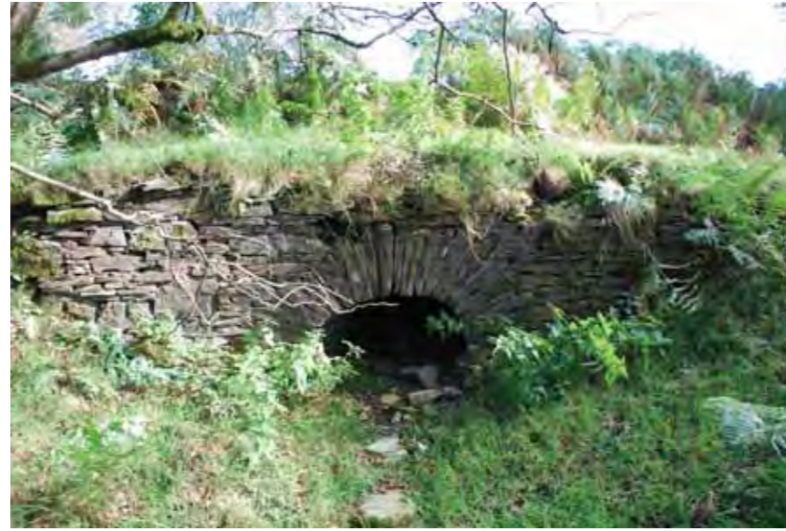
PDT4 - Bridge on Site access trackway
