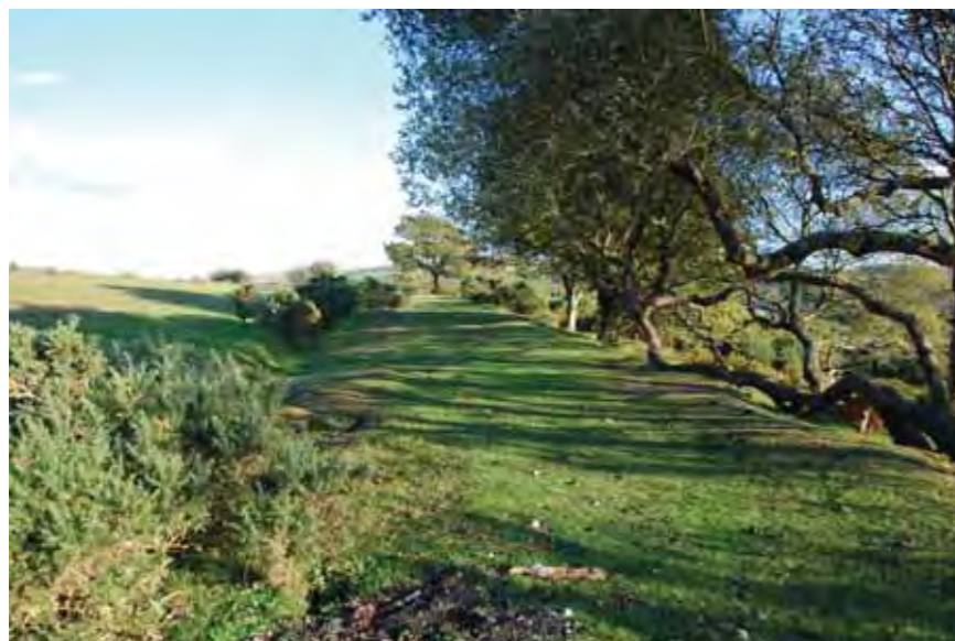
PDR3 - Embankment sits above surrounding ground level
